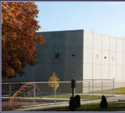
Oak Park Elementary School, Des Moines, Iowa
